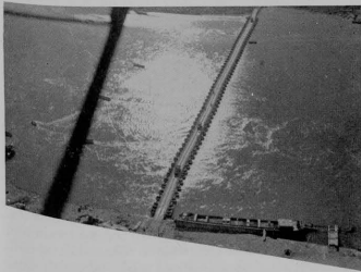
Vehicles cross Rhine on heavy pontoon bridge constructed by Corps Engineers at Kripp-Linz.
